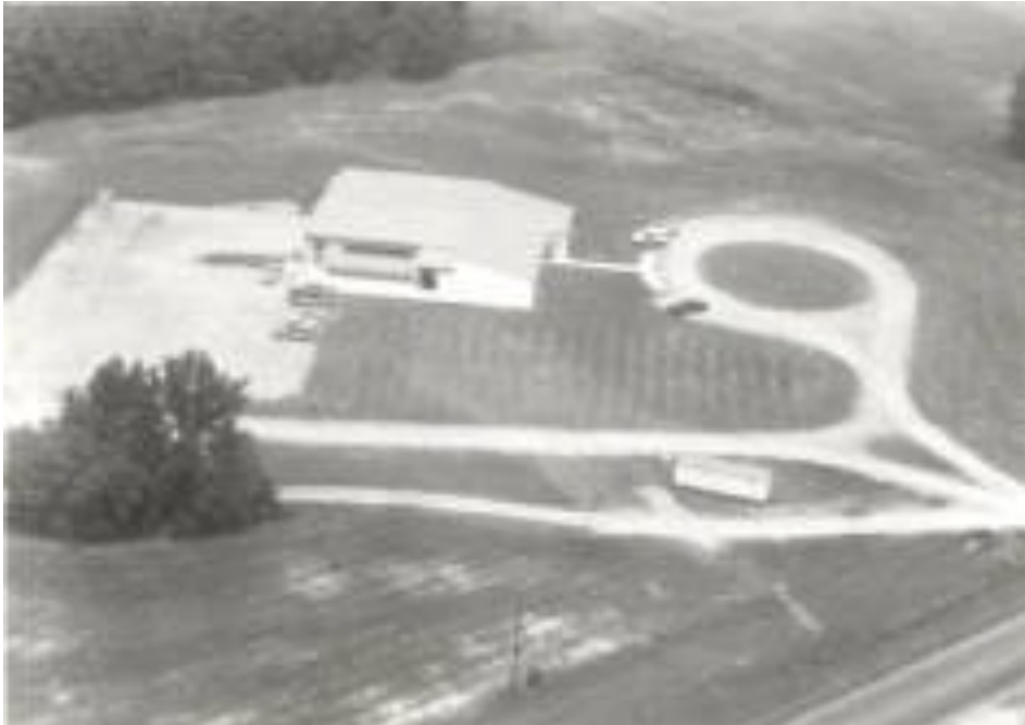
Aerial photograph of the first phase of the Harnett County Campus
